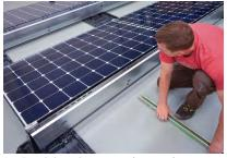
Position Strut under and near center of PV module in line with center slots on Wind Deflector. Position Strut throughout the array as shown on array design layout.
