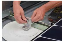
9. Attach L-Bracket 2 to L-Bracket 10. Attach L-Bracket 2 to Strut. 1 by butting flat sides and bolting together. Use included L-Bracket Bolt to secure two L-Feet together. Tighten Bolt to 14 ft-lbs.
