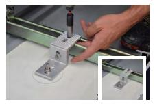
8. Attach L-Bracket 1 to Roof Attachment. Place long side of L-Bracket on Roof Attachment and secure L-Bracket 1 to Roof Attachment with Bolt. Tighten Bolt to 14 ft-lbs.
