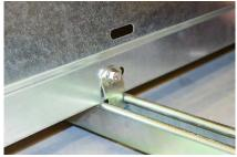
7. Using Strut Strap Components shown, attach North row Strut Strap to Wind Deflector and Strut. Place Bolt behind Wind Deflector and bottom of Strut Strap in Strut channel. Tighten Bolt to 14 ft-lbs.
