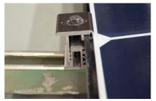
6. Assemble Clamp components as shown. Attach South row Module Clamps onto Strut and Modules. Place Strut Nut into Strut channel. Slide Clamp to Module Frame. Tighten Bolt to 14 ft-lbs.
