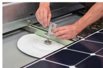
8. Attach L-Bracket 1 to Roof Attachment. Place short side of L-Bracket on Roof Attachment and secure L-Bracket 1 to Roof Attachment with Bolt. Tighten Bolt to 14 ft-lbs.
